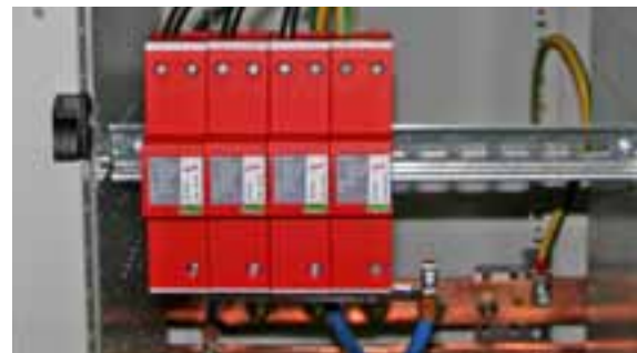
Figure 7 Coordinated class I surge arrester
