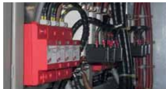
Figure 8 Protection of the rotor winding of the generator ("Neptune" circuit)
