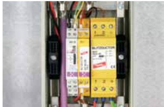
Figure 10 Protection of the weather station (anemometer)
