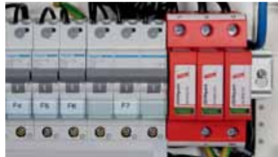
Figure 6 Modular class II surge arrester for protecting 230/400 V power supply systems
